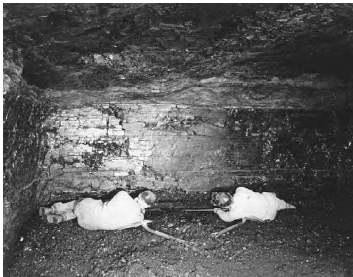
FIGURE 29.1 Miners undercutting a coal face prior to mechanization. (From National Archives. With permission.)
